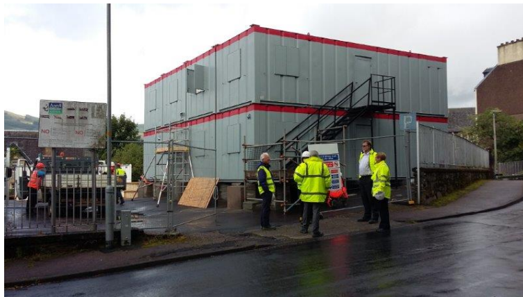
Site offices being installed in car park off Kirk Street
