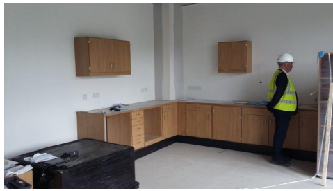
Staffroom awaiting white goods to be installed
