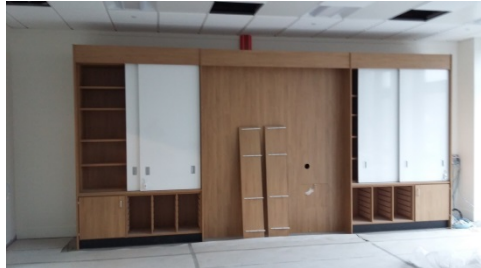
Teaching walls installed awaiting installation of interactive screen
