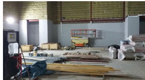
Sports hall – acoustic paneling, retractable seating and flooring to be installed
