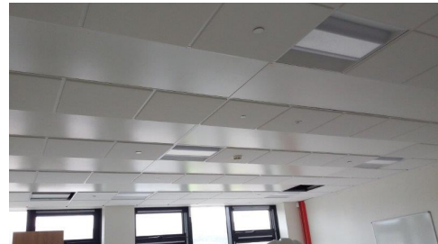
Ceiling installations mainly complete with integrated radiant panels
