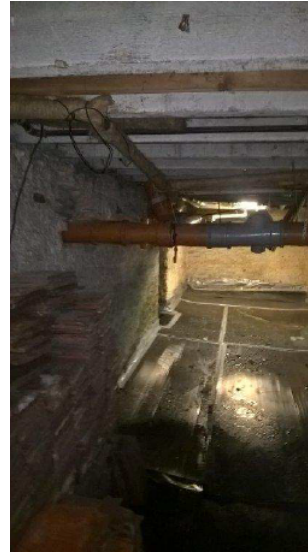
Encapsulation works to solum of West Wing
