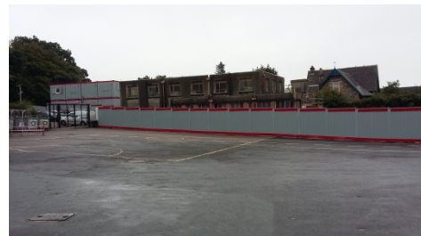
Site hoarding to main playground area
