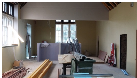
Internal works ongoing in 1881 building
