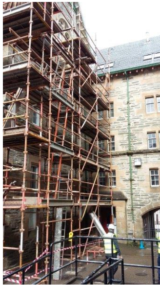
Scaffolding to West elevation at the existing pend entrance to the school from Hillfoot Street
