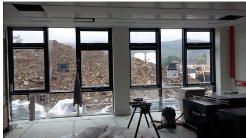
Window installations in classrooms
