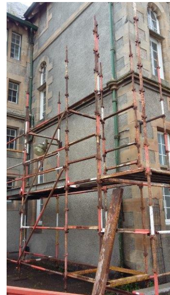
Scaffolding being erected on Hillfoot St elevation of West Wing
