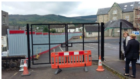
New pedestrian and vehicular access gates on Kirn Street
