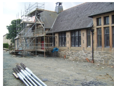
External works to 1881 building nearing completion. Groundworks to commence
