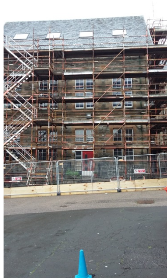
Scaffolding being erected to West Wing (rear elevation)
